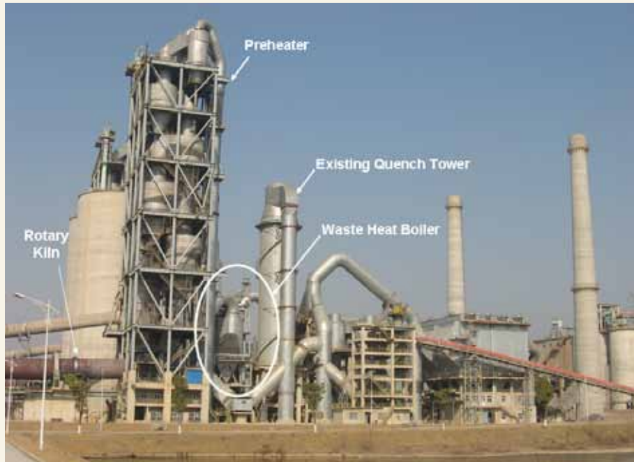
Figure 5: Preheater Waste Heat Boiler
