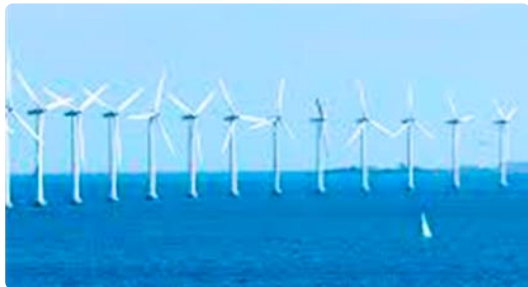
Wind turbines installed with use of ECONcrete 67
