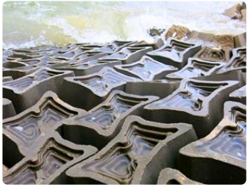
ECONcrete used in a coastal fortification structure 66
