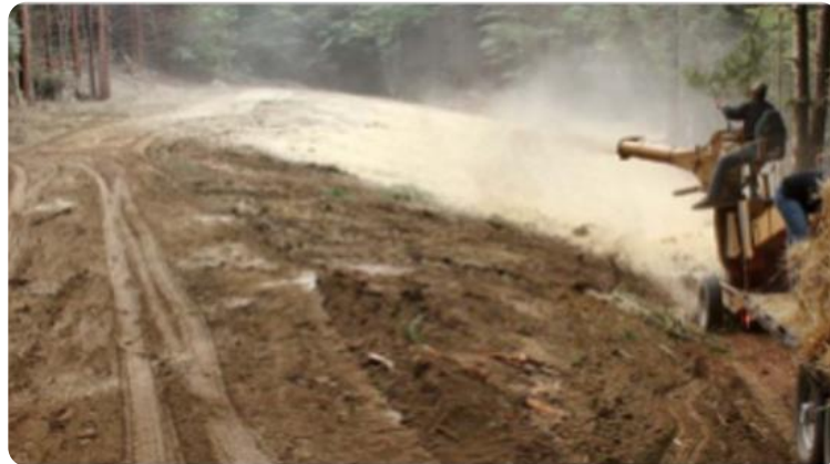
Seeding and mulching (suing a straw blower) of an exposed area from a decommissioned road
