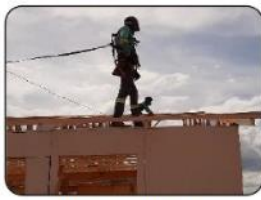
Work at height
